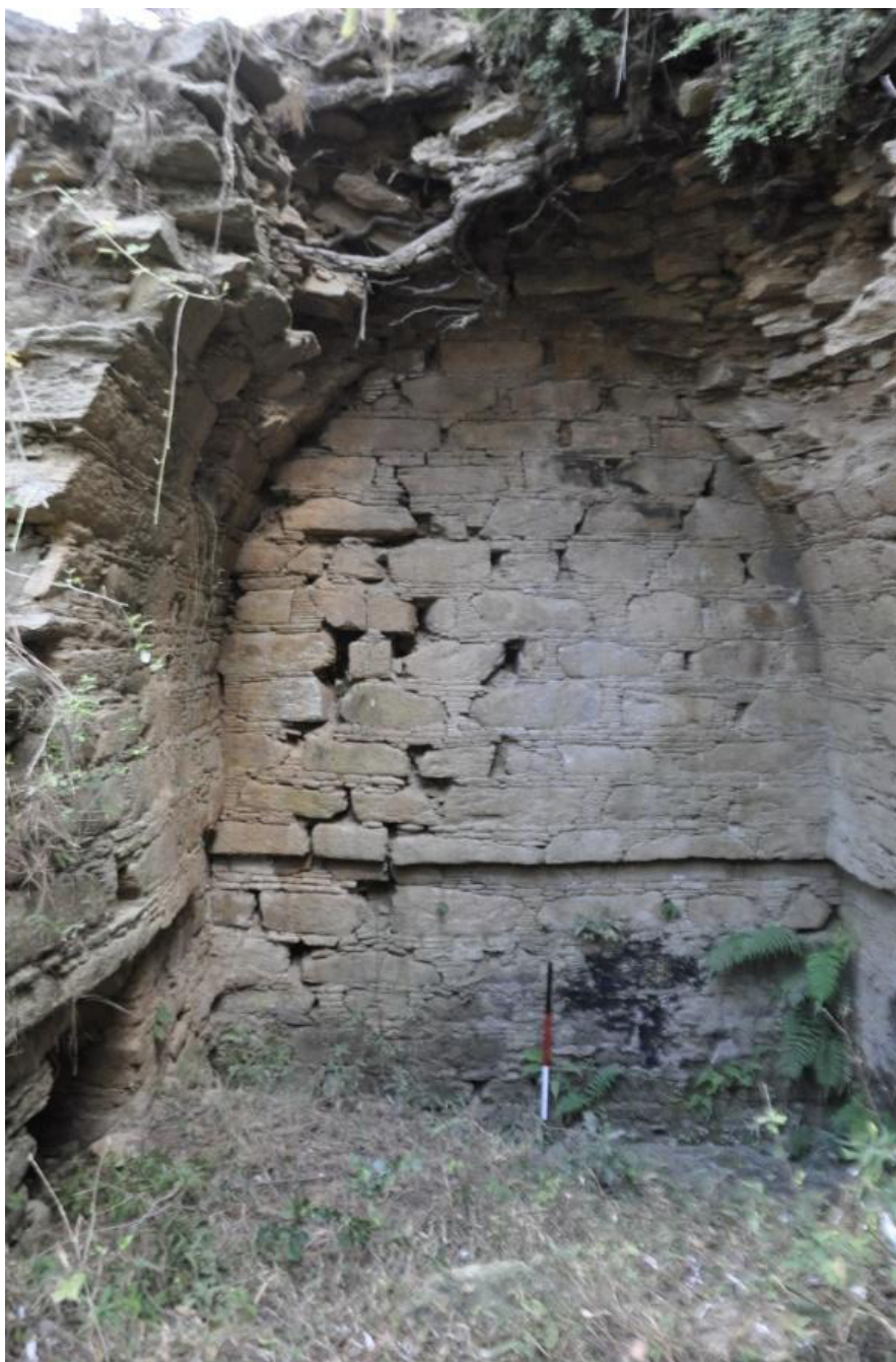
Fig. 20 - Corbelled Roof and Double-Storey Structure at Rāmāñrai.
