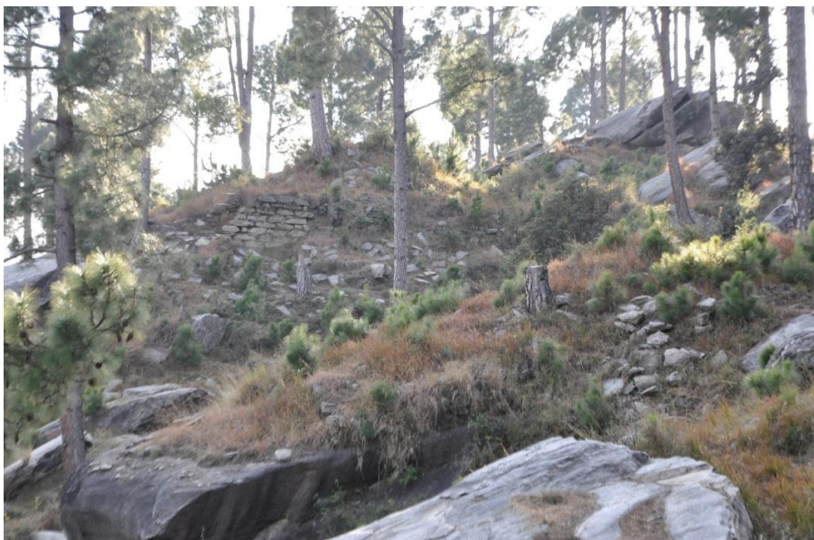
Fig. 19 - One of the embankment to support the structures and channel the floods.
