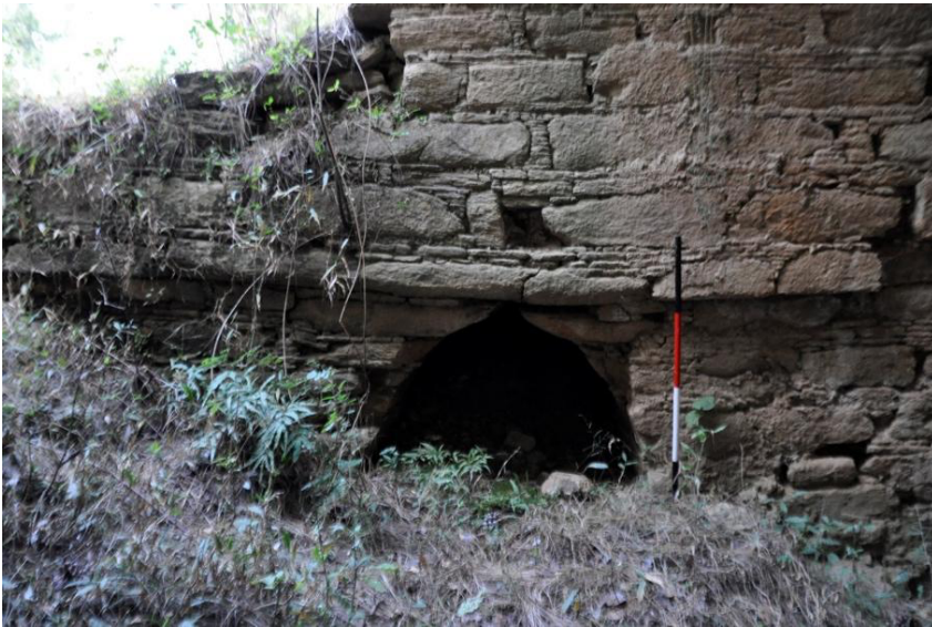
Fig. 21 - Arched doorway to the corbelled roofed double-storey structure.
