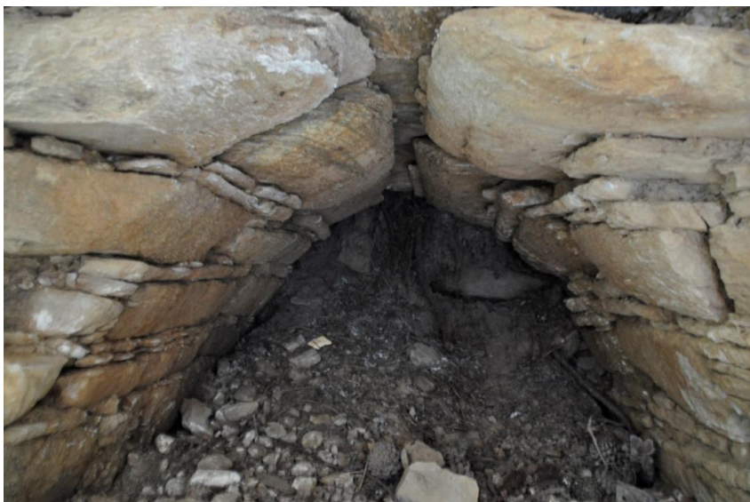
Fig. 16 - Roof of a Channeled Spring at Rāmāñrai.
