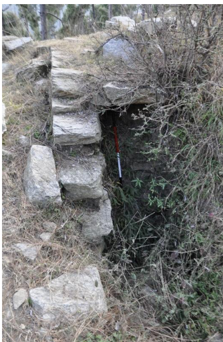
Fig. 17 - One of the roofed channels of water.
