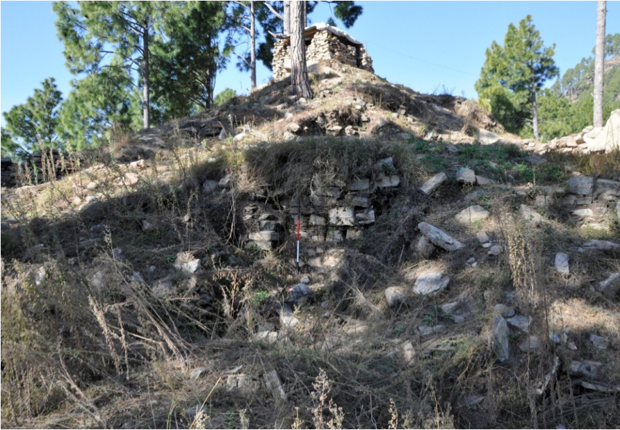
Fig. 15 - Parts of the base and drum of Juro Stupa.
