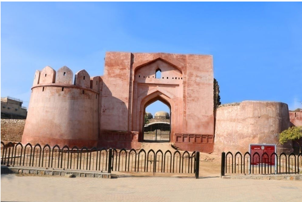
Fig 2 - Façade of Rewat Fort.
