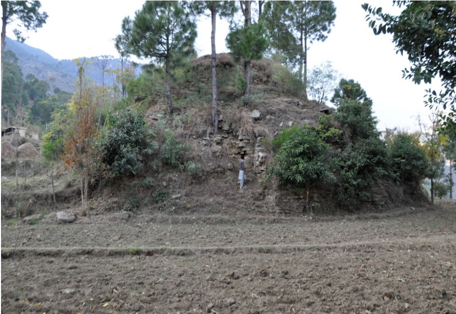
Fig. 3 - Kafero Dherai Stupa (Showing Flight of Steps).
