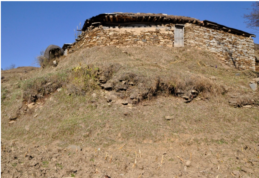
Fig. 14 - Exposed Structures at Ilam Village Site.
