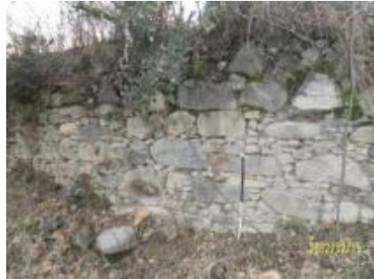
Fig. 12 - Portion of the wall, WGB (S-III).
