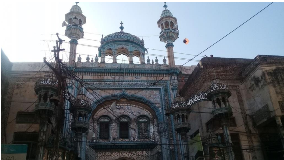
Fig. 2 - Main Entrance Gate of Markazi Jamia Masjid (Photo by Mujeeb Ahmad).
