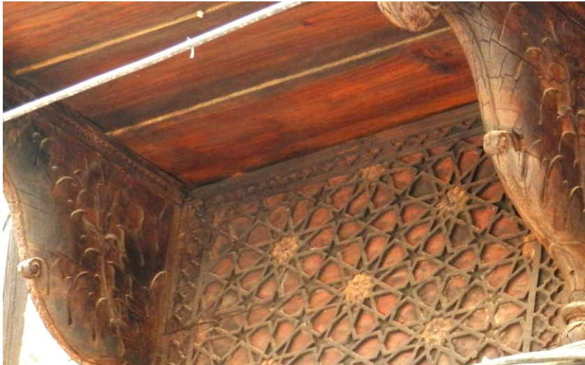
Fig. 3 - Stellar Motif under the Eave of a Balcony, near Wazīr Khān Mosque (Photo by the Author).
