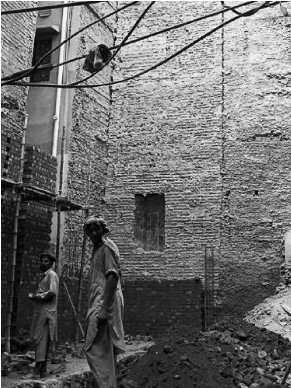
Fig. 11 - A construction site showing the use of multiple types of bricks.
