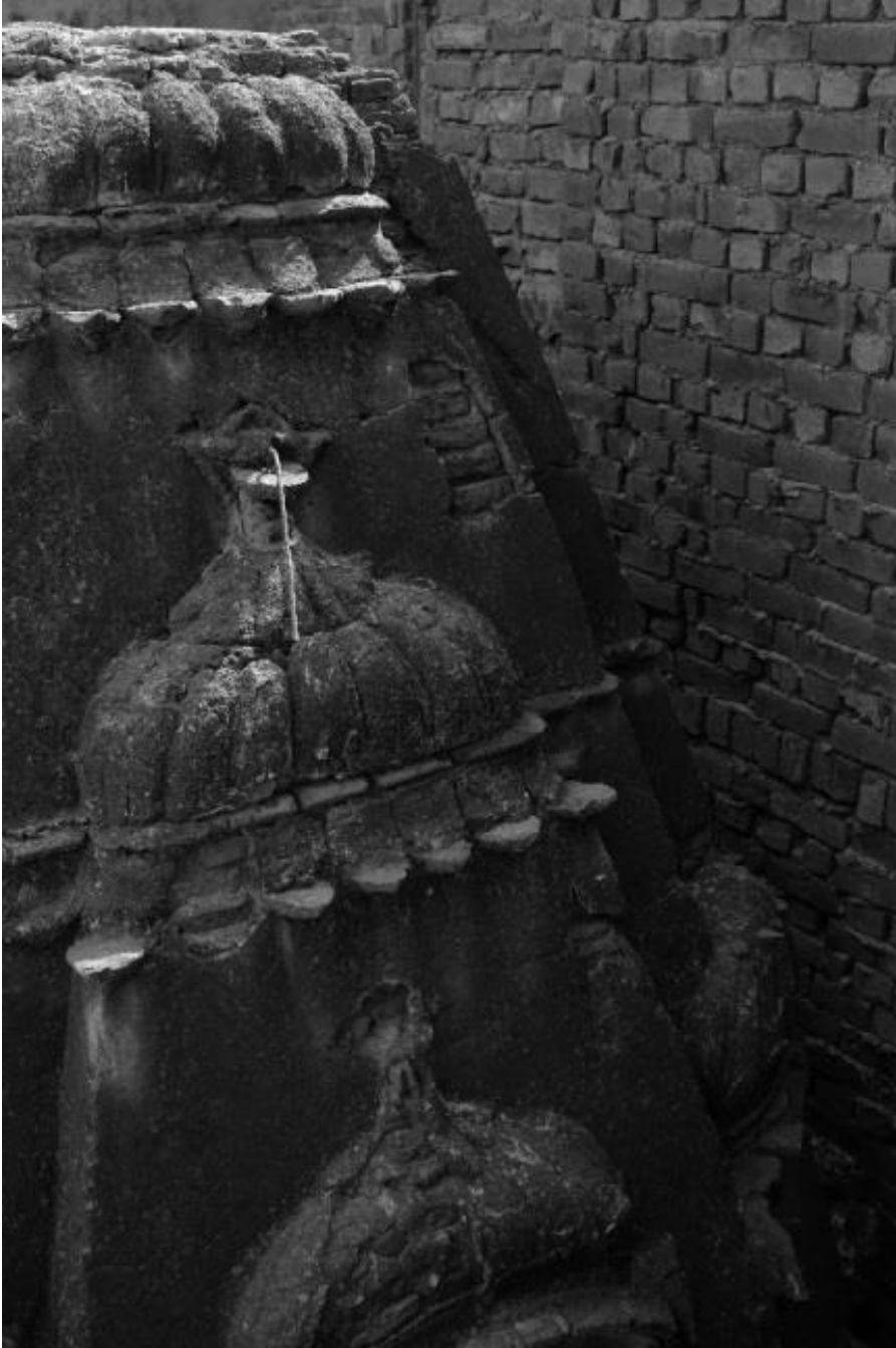
Fig. 5 - View of shikara from roof of opposite building.
