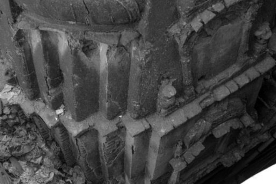
Fig. 6 - View from above.
