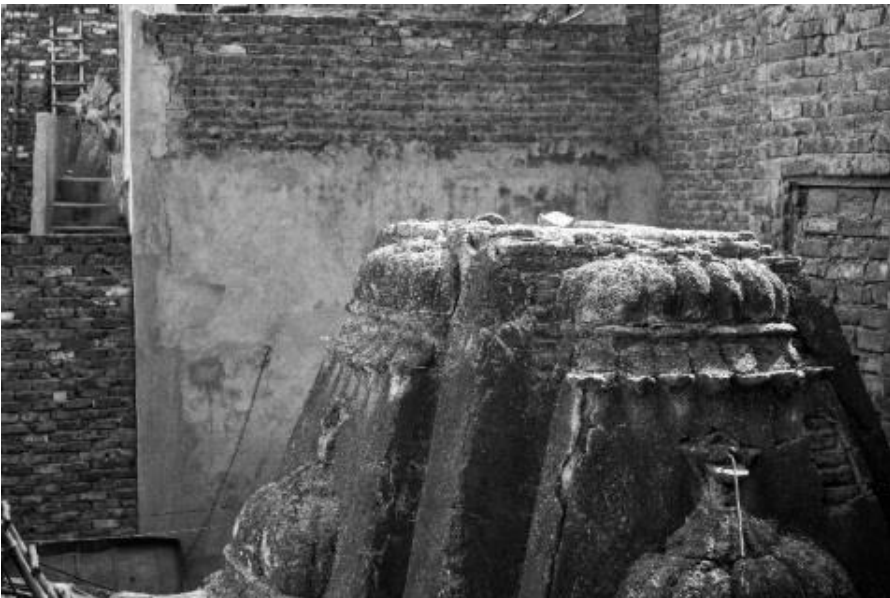
Fig. 7 - View across, showing remains of another shikara in background.
