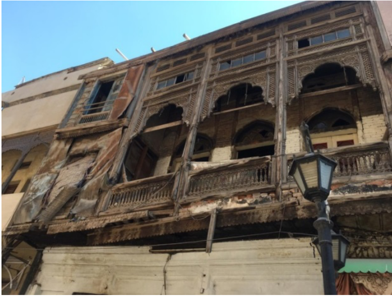
Fig. 11 - Old Building on Heritage Trail (Photo by AGK).
