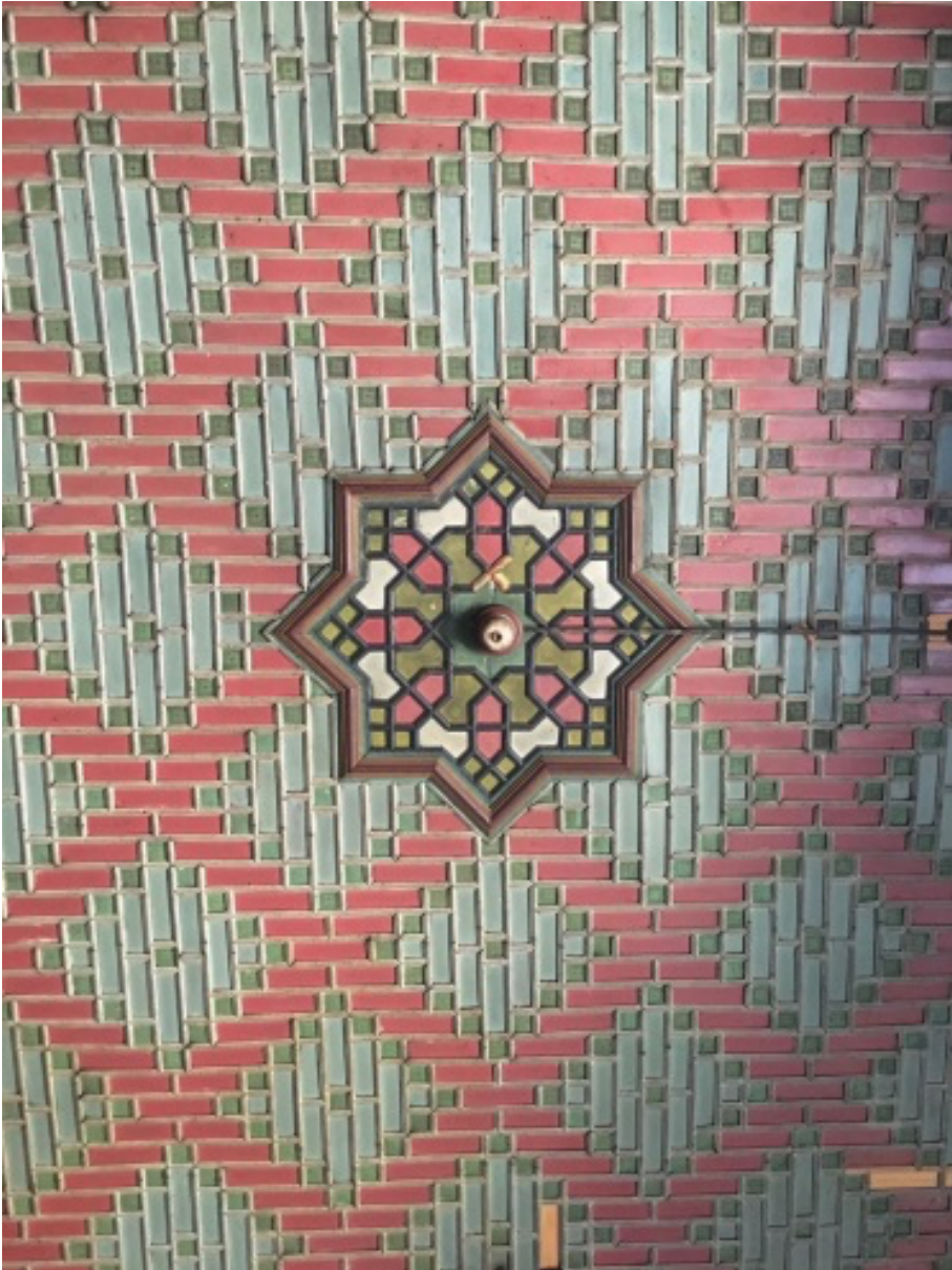
Fig. 7 - Ceiling in Sethi House Complex (Photo by AGK).
