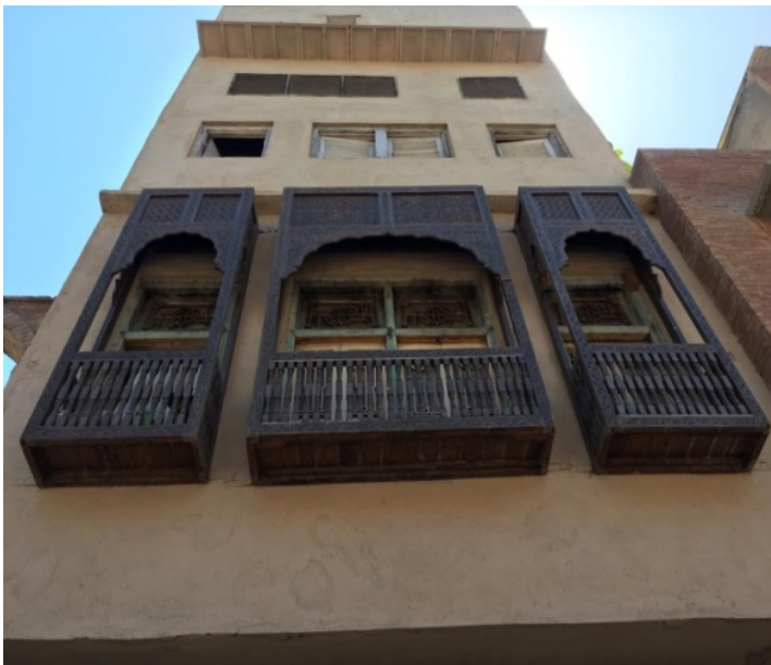
Fig. 10 - Wooden facades on buildings (Photo by AGK).
