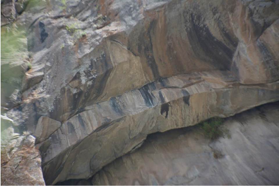
Fig. 7 - Details of top arch of Rock Cut.
