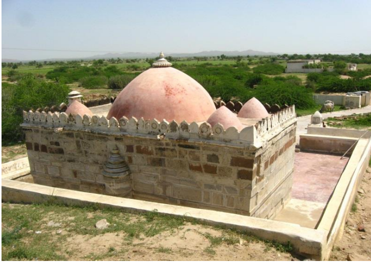
Pl. I: Bodhesar: A view of Mosque from the south-west corner
