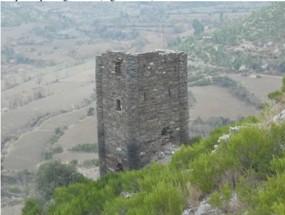
Fig. 7- The most intact watchtower showing platform, windows on 2 nd and 3 rd floors and the arrow-slits, site 111, Charat Pass, district Malakand Agency.
