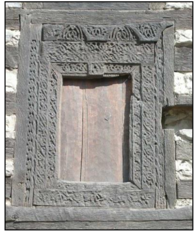
Fig. 9: Western casement to the first floor of watch tower.
