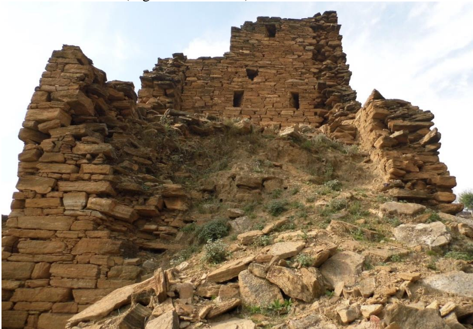
Fig. 8- Showing the filled platform, arrow-slits, beam slot and a window on the upper extreme left side, site 153, Tauda Cheena, Lower Dir.
