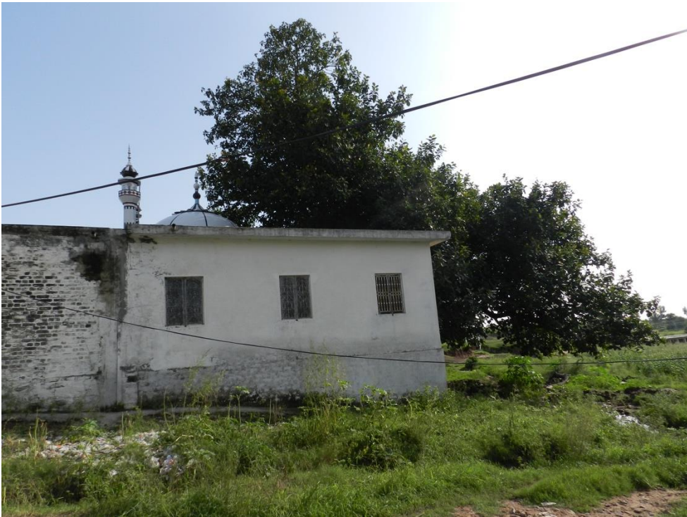
Fig. 9 - Akbari Masjid after the renovation (1994).
