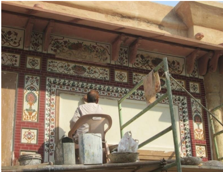
Fig. 12 - The motif or floral design is filled with the required colors as per original design.
