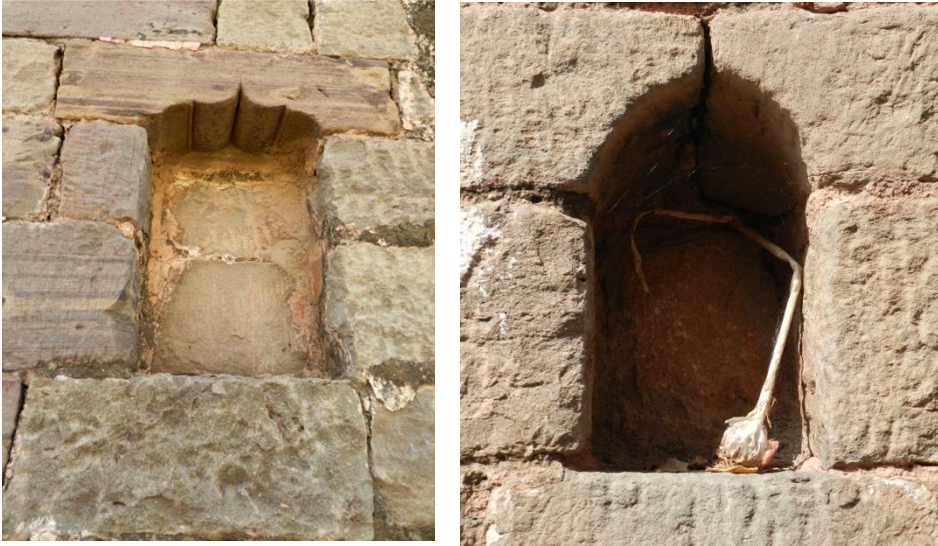
Figs. 36-37 - Niches at the entrances of houses, shaped with skillfully chiseled stone.
