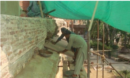
Fig. 8 - Restoration and placement of sandstone eaves.
