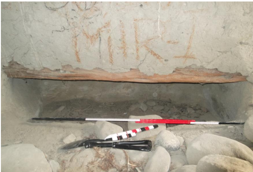
Pl. 20 - Ɖom-rā: current condition of preservation of above side chamber or niche.
