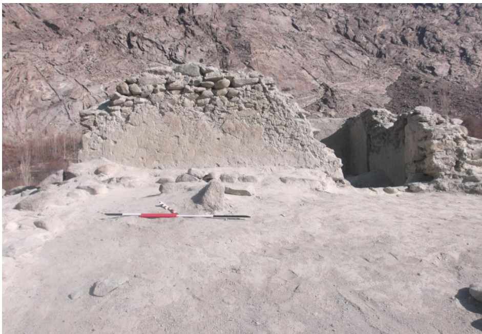
Pl. 17 - Dom-rā: façade, present condition of preservation.
