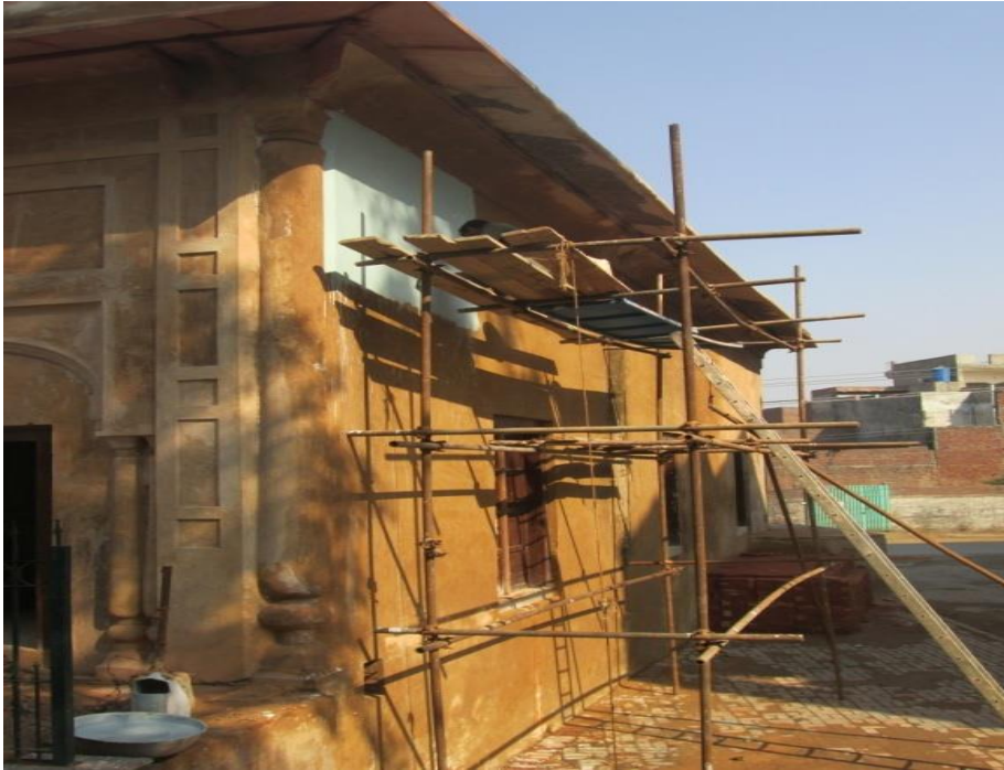
Fig. 10 - Application of course kankar lime mortar as a base coat.
