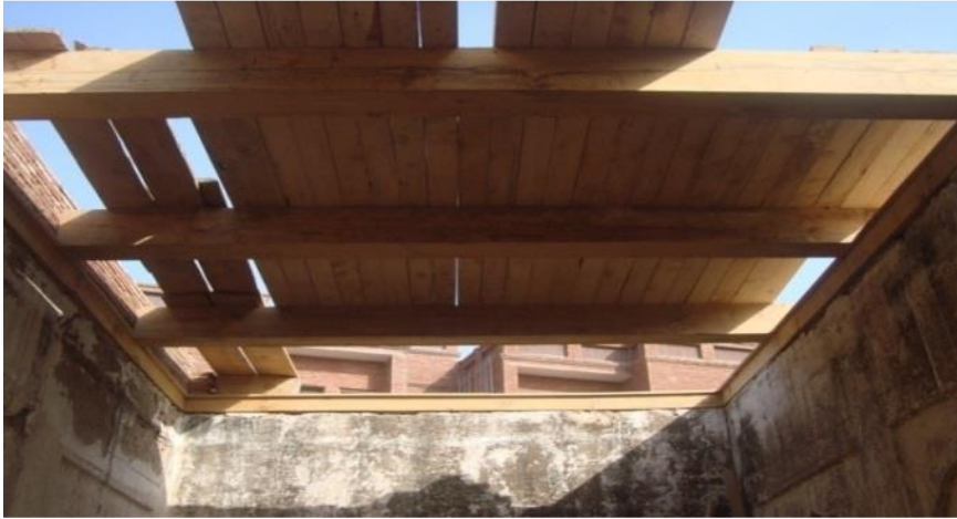
Fig.7 - Placement of deodar wooden beams and planks for roofing.
