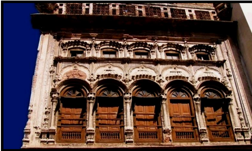
1b. Windows and ventilators of upper storey, Bhabra Bazaar , Rawalpindi
