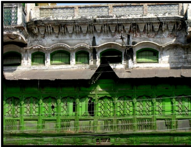
4a. Wooden Balcony: Raja Bazaar , Rawalpindi
