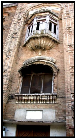
5a. Upper storey windows in Daultala town
