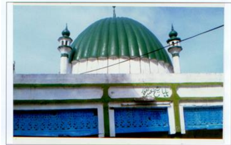
Pl.-II Shaikh Mahallah: Close up view of Pl.-I
