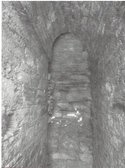
Pl. 5: Balo-Kale Gumbat vihāra, the northern side ambulatory detail of the corbelled ceiling (Meister & Olivieri 2012: fig. 9)
