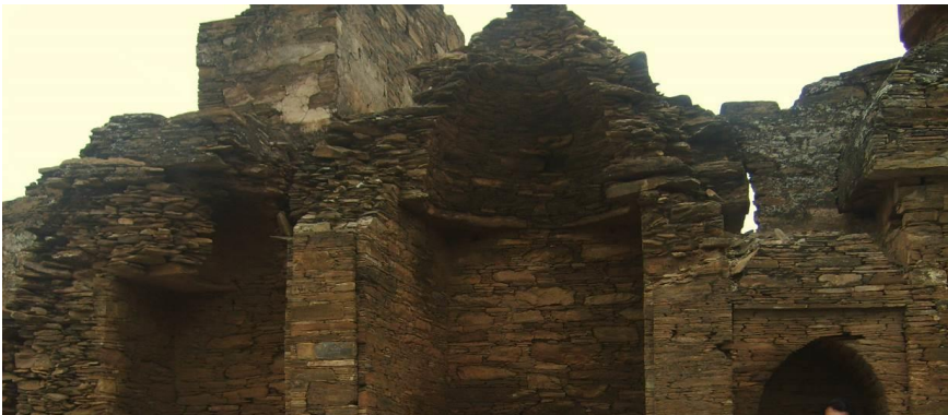
Pl. 9: A chapel to the south of the main stūpa at Takht-i-Bhai showing corner pendentives
