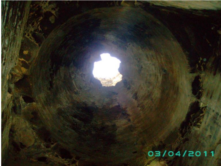
Pl. 10: Balo- Kale Gumbat: Interior detail of the double dome ceiling (before conservation)
