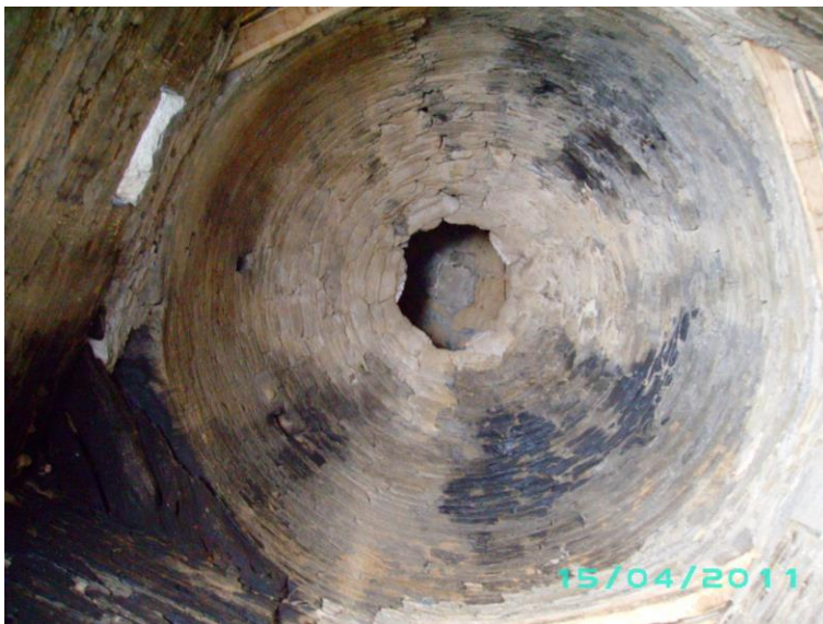
Pl. 11: Balo-Kale Gumbat: Interior detail of the double dome ceiling (after conservation).
