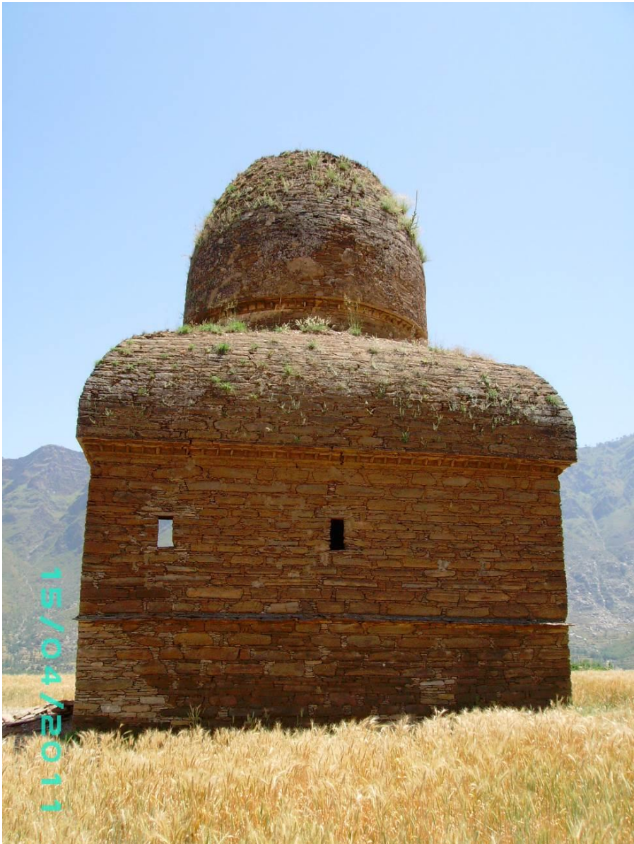
Pl. 3: Balo-Kale Gumbat: General view from the southern side
