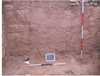
Fig 22: Mud plaster preserved on interior wall of Cell 4
