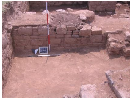
Fig 32: Interior of eastern wall of Cell 6
